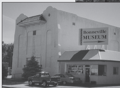
Masonic Temple as it existed prior to its acquisition by the museum.
